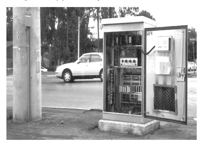
The older NEMA standard for traffic signal control equipment is known as the TS-1 standard while the newer standard is known as the TS-2 standard. The first version of the TS-1 standard was introduced in 1975 and the first version of the TS-2 standard was introduced in 1998. Prior to 1975, there was no industry standard for traffic control equipment and no interchangeability amongst controller manufacturers.
