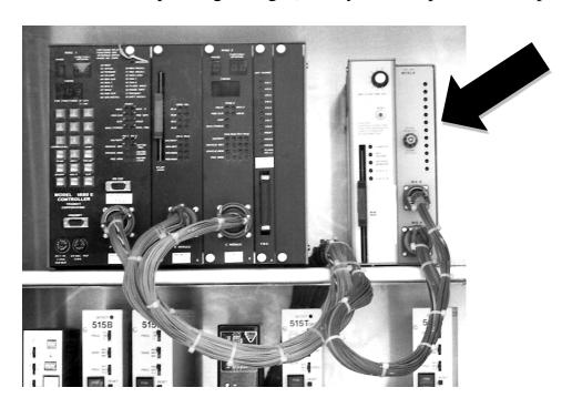
If the conflict monitor detects that two conflicting phases (phases that control conflicting vehicle movements) are active at the same time, the monitor will immediately place the intersection into latched flashing operation. A phase is considered to be active if it has either a green, yellow, or walk indication. Latched flashing operation is flashing operation that will continue until the conflict monitor's reset button is activated.
