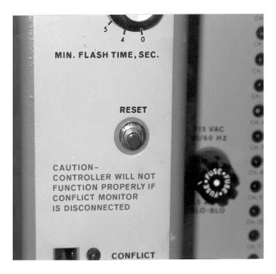
The reset switch should only be used when the problem which caused the conflict has been identified and corrected, or during conflict monitor testing.
