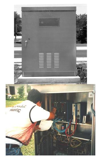
The field wires from the cabinet run through conduit that is encased in the cabinet foundation. Larger cabinets are typically ground mounted because of their considerable size and weight. Unless extenuating circumstances prevent it, the cabinet door should open away from the intersection. This allows the technician to easily monitor signal head indications and traffic behavior while, at the same time, observing the operation of the controller and detector units located within the cabinet.
