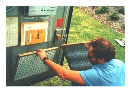
The cabinet cannot be completely sealed from water since air input vents are needed for the air circulation system to work. Consequently, if the cabinet is located close to the road and the door opens toward the road, passing vehicles may splash puddled water through the air input vents and into the cabinet. This is another reason to orient the cabinet so that the door opens away from the intersection.
